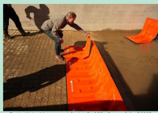
Test in Water Management Center, Roskilde, Denmark April 2025
